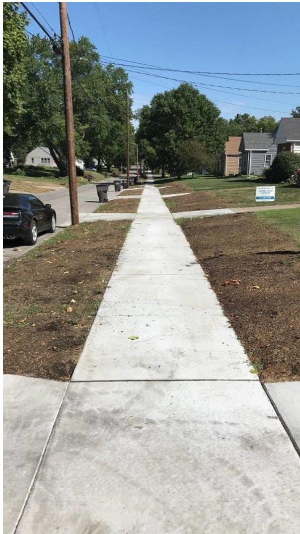
Sidewalk on 45 th Street
